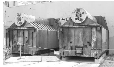
Boilers before and after stack removal
