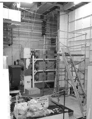
The XCR will be cleaned out to provide access to PPC below
