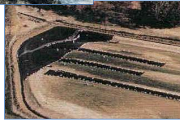
Geomembrane cover installation
