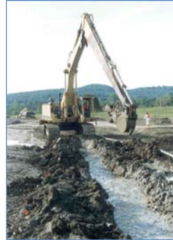
Subsurface barrier wall installation
