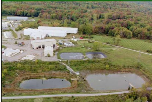
LLW Treatment System includes treatment building, underground tanks and lagoons
