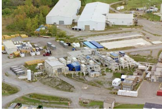
Aerial view of the underground radioactive waste tank area
