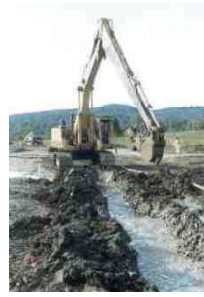
Slurry Wall Construction
