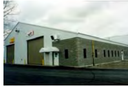
Exterior of Lag Storage Area 4, one of the facilities used to process and package waste and prepare it for shipment off site
