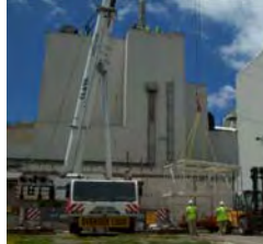
XC-3 enclosure installation in preparation for vessel removal
