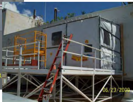
Installation of platform and enclosure atop the Main Plant Office Building for Hot Acid Cell vessel removal
