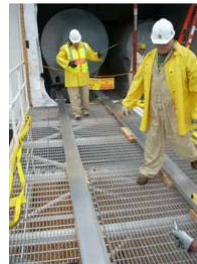
Workers prepare to remove the vessels
