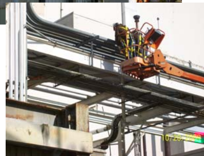
Electrical equipment isolations and piping removal began in Oct
