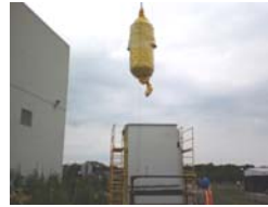
Vessel being removed from XC-3
