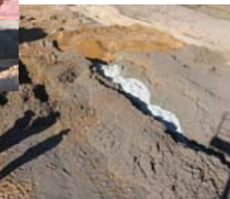
Section of test trench
