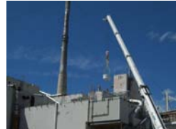
Crane lift of waste containers from PMCRE
