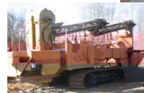
Trencher in operation
