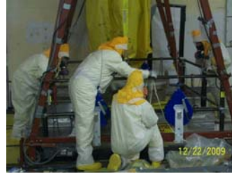
Separator being removed from XC-3
