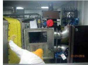
Installation of adaptor for T&VDS vent lines
