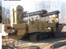
Trencher in operation
