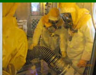
Temporary ventilation ducting placed into Tank 8D-1 M-7 Riser
