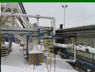
Temporary lines will provide ventilation while old lines are replaced
