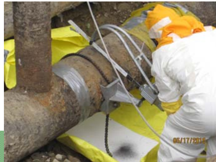
Section of underground 16" ventilation header removed
