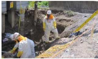
Removal of 16" underground ventilation pipe
