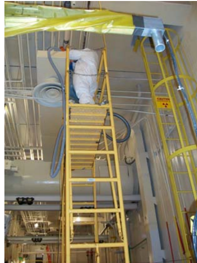
Asbestos removal completed in the General Operating Aisle
