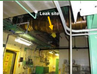
Area where contaminated duct was remediated
