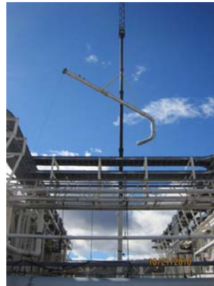
Ductwork installation
