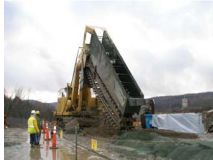
Completion of the Permeable Treatment Wall
