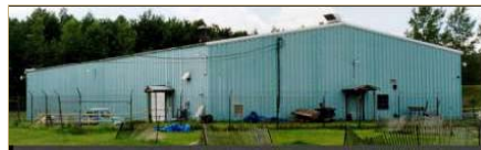
Bulk Storage Warehouse
