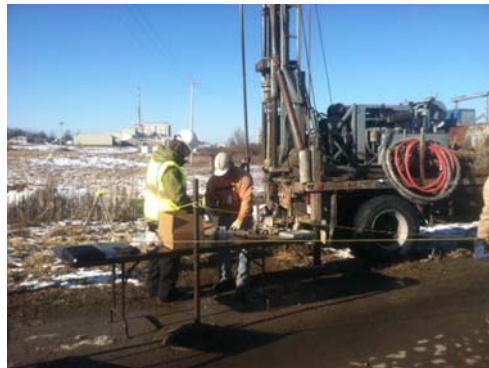
Boring of Sub-Surface Soils
