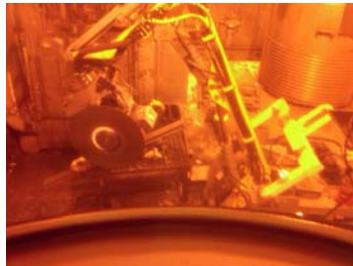
BROKK cutting SBS
