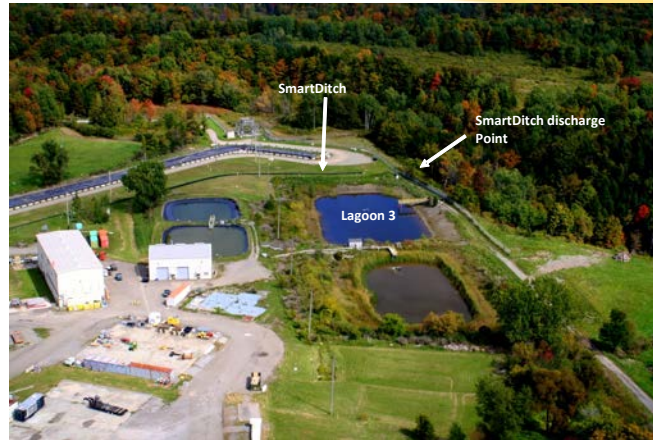
Aerial photo of lagoon system showing location of Smart Ditch® and current Smart Ditch® discharge (goes under road and discharges at top of embankment)
