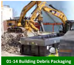
01-14 Building Debris Packaging
