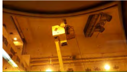
Fixative Application in Vitrification Cell Ceiling
