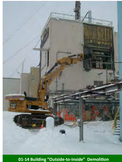
01-14 Building "Outside-to-Inside" Demolition
