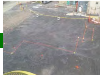
01-14 Building at Start and Completion of Demolition
