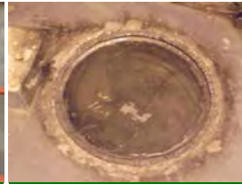
Utility Lines Sealed Shut
