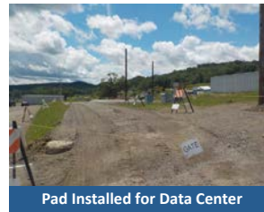
Pad Installed for Data Center
