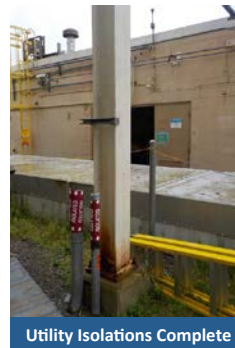
Utility Isolations Complete
