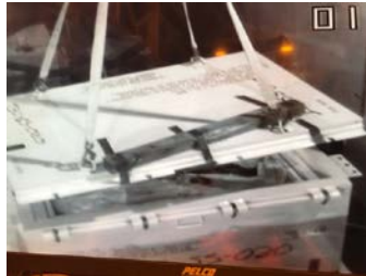
Non-HLW Drum Packaging in the Chemical Process Cell
