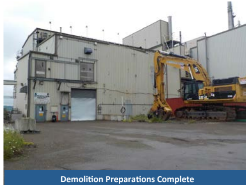
Demolition Preparations Complete
