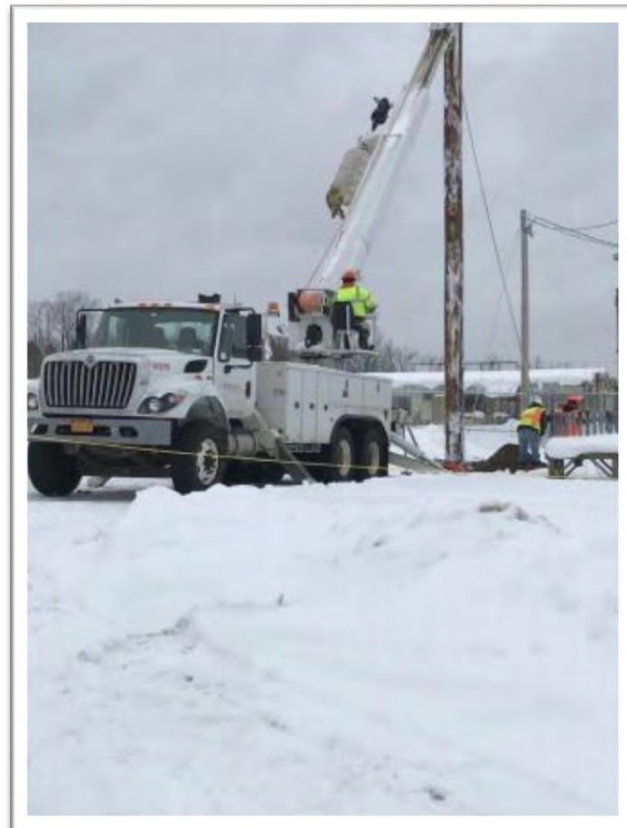
Pole being installed for new electrical substation
