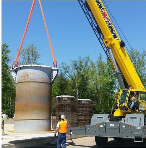
CH2M HILL BWXT West Valley workers place a vertical storage cask liner on a construction pad.
