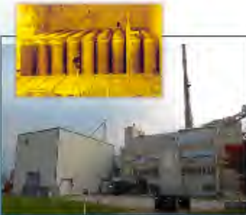
Canisters Stored Inside Main Plant
