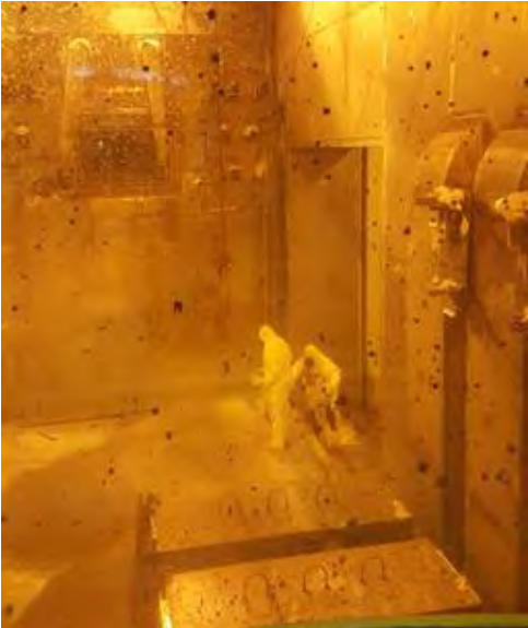
Workers perform some pre-demolition procedures in the vitrification building. (CHBWV)
