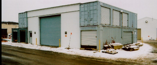
Maintenance Storage Area
