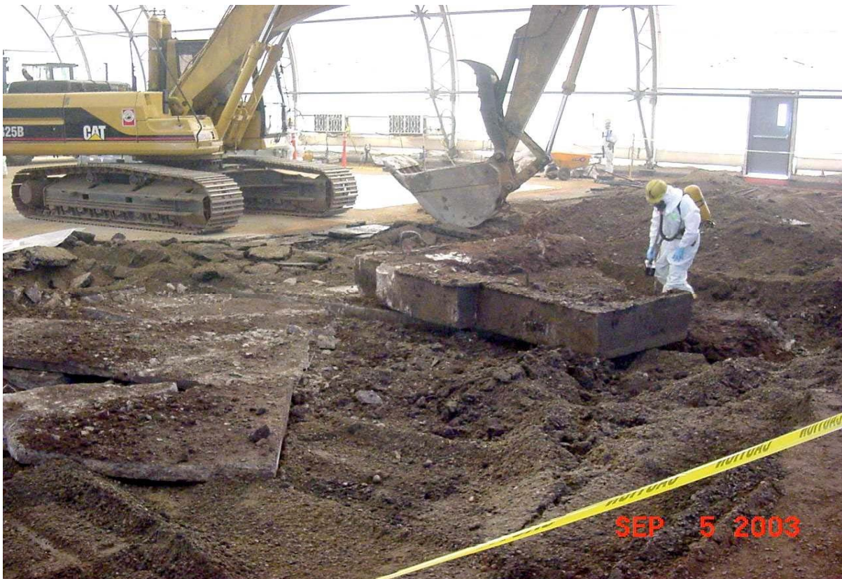
903 Pad demolition inside tent, 2003
