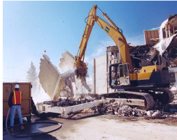
Demolition activities at Rocky Flats
