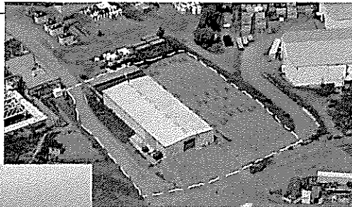
Lag Storage Building Before (above)
