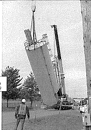
CSS Silo – Being removed (right) and size-reduced (left)
