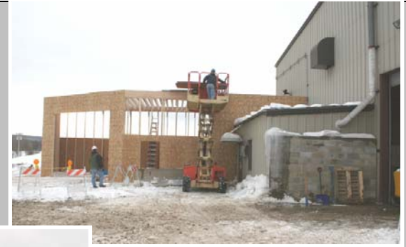
Package finalization area under construction
