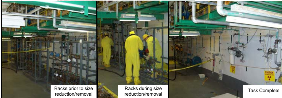
Main Plant Upper Extraction Aisle racks and piping removal
