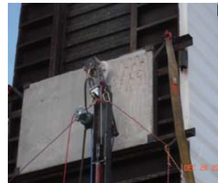
Deploying remote-operated scabbler equipment and tooling (above) on the Off-Gas Cell walls (below) will reduce dose rates in the cell.
