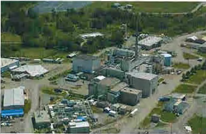
Credit: Copyright 2006 James Cavanaugh The West Valley Demonstration Project, New York
