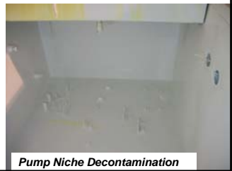
Pump Niche Decontamination
