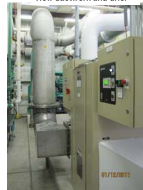
04/29/2010 22:59 New ductwork and drier
