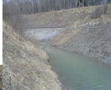
Close-up view of the canal
