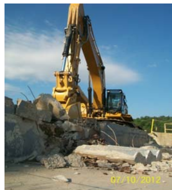
Demolition of the Warehouse pad
