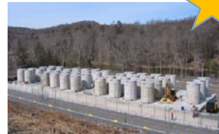
High Level Waste Canister Storage Relocation Procurement
