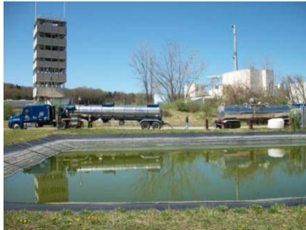
Sludge removal in Sewage Treatment Plant and Equalization Basin 100% Complete (1.3M Gallons)
