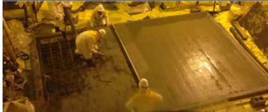
Completed EDR Soaking Pit Cap Installation (Before/After)
