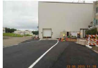
Completed Cask Transfer Pad
