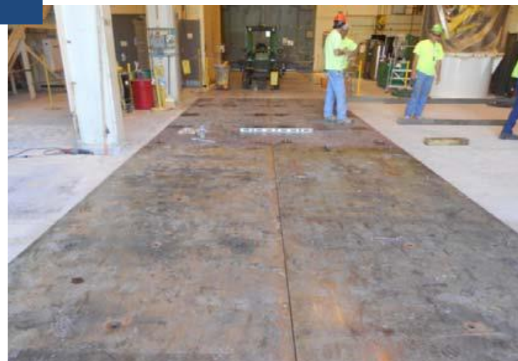
Balance of LIF Runway Floor Plating was Installed (Left) and Grouting Beneath the Plates (Right) was Completed
