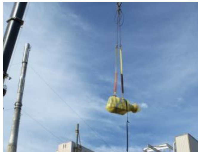
Motor Gear Reducer Removal
