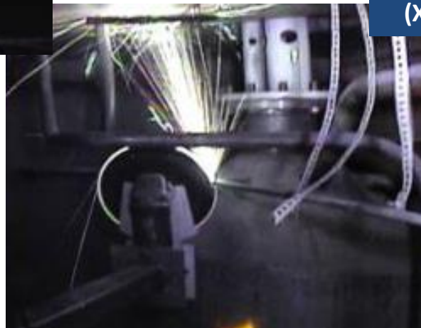
Liquid Waste Cell Pipe Removal
