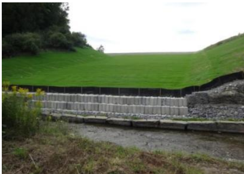
Lake 1 Spillway Before the Storm
