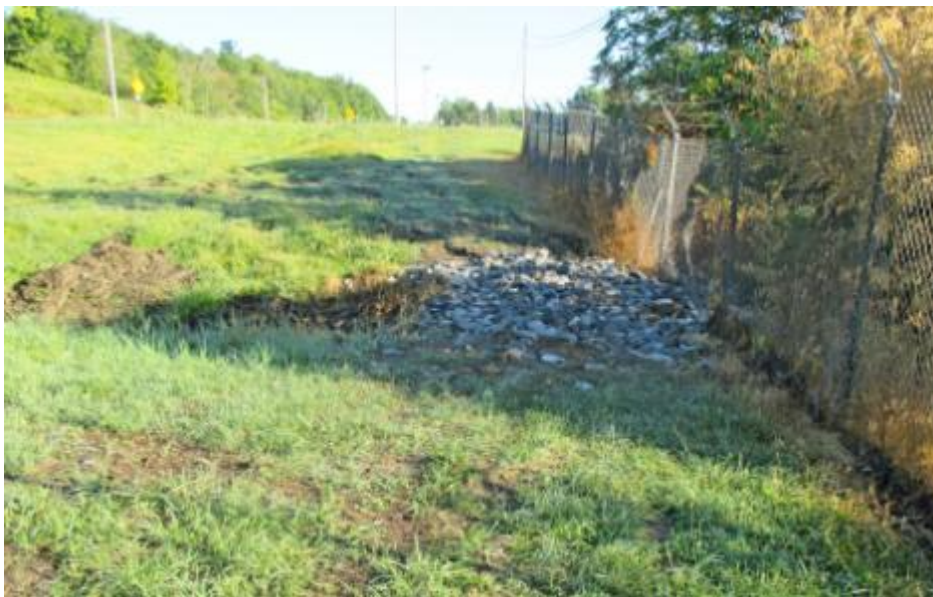
CHBWV Repaired the Gap in the Fence on June 17 with 54 Tons of Surge Stone
