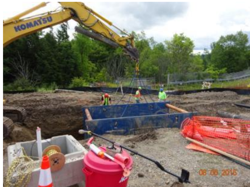
Progress Continued with the Storm Water Outfall Relocation Project
