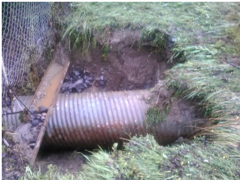
CHBWV Repaired the Gap in the Fence on June 17 with 54 Tons of Surge Stone
