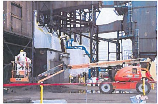
A crew is doing asbestos work at the Portsmouth Gaseous Diffusion Plant in Piketon.
