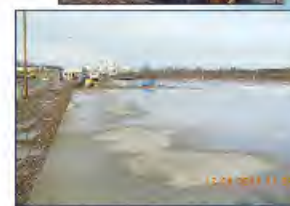
Five separate concrete placements and more than 300 concrete delivery trucks involved in completing the HLW Storage Pad and Approach Apron.
