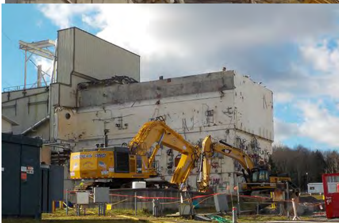
Workers tear down portions of the Vitrification Facility with the least radiological contamination in the first phase of demolition.
