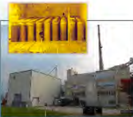
Canisters Stored Inside Main Plant
