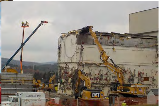
Workers tear down portions of the Vitrification Facility with the least radiological contamination in the first phase of demolition.
