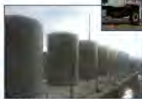
The First 8 Concrete Vertical Storage Casks
