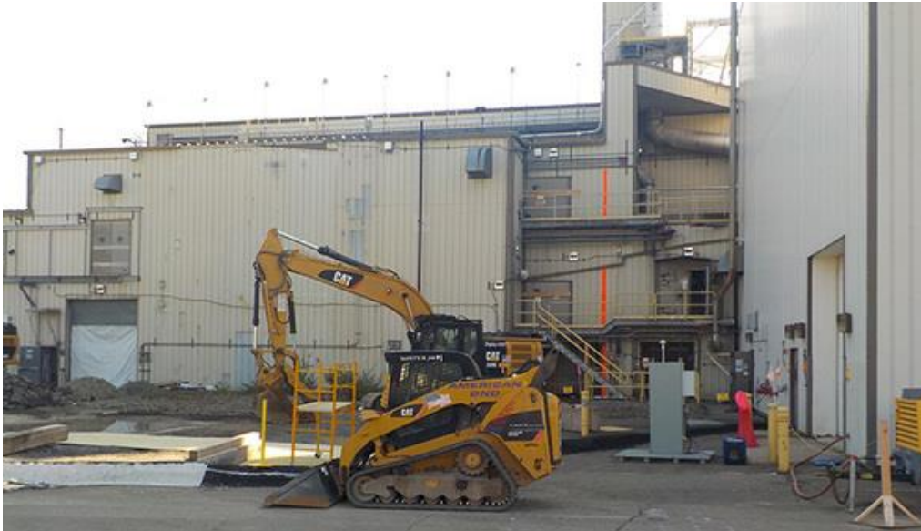
Demolition equipment is staged in front of the Vitrification Facility.
