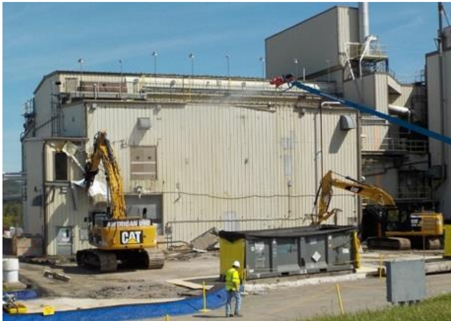
Demolition underway at the WVDP vitrification facility (Image: DOE)
