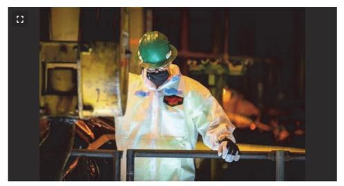
Paducah site worker Brandon signals a crane operator to lower a motor from the C-333 Process Building's cell floor to the truck alley for removal. The work was done to support the future construction of a Material Sizing Area in the building, which will be used to downsize large components for disposal.
