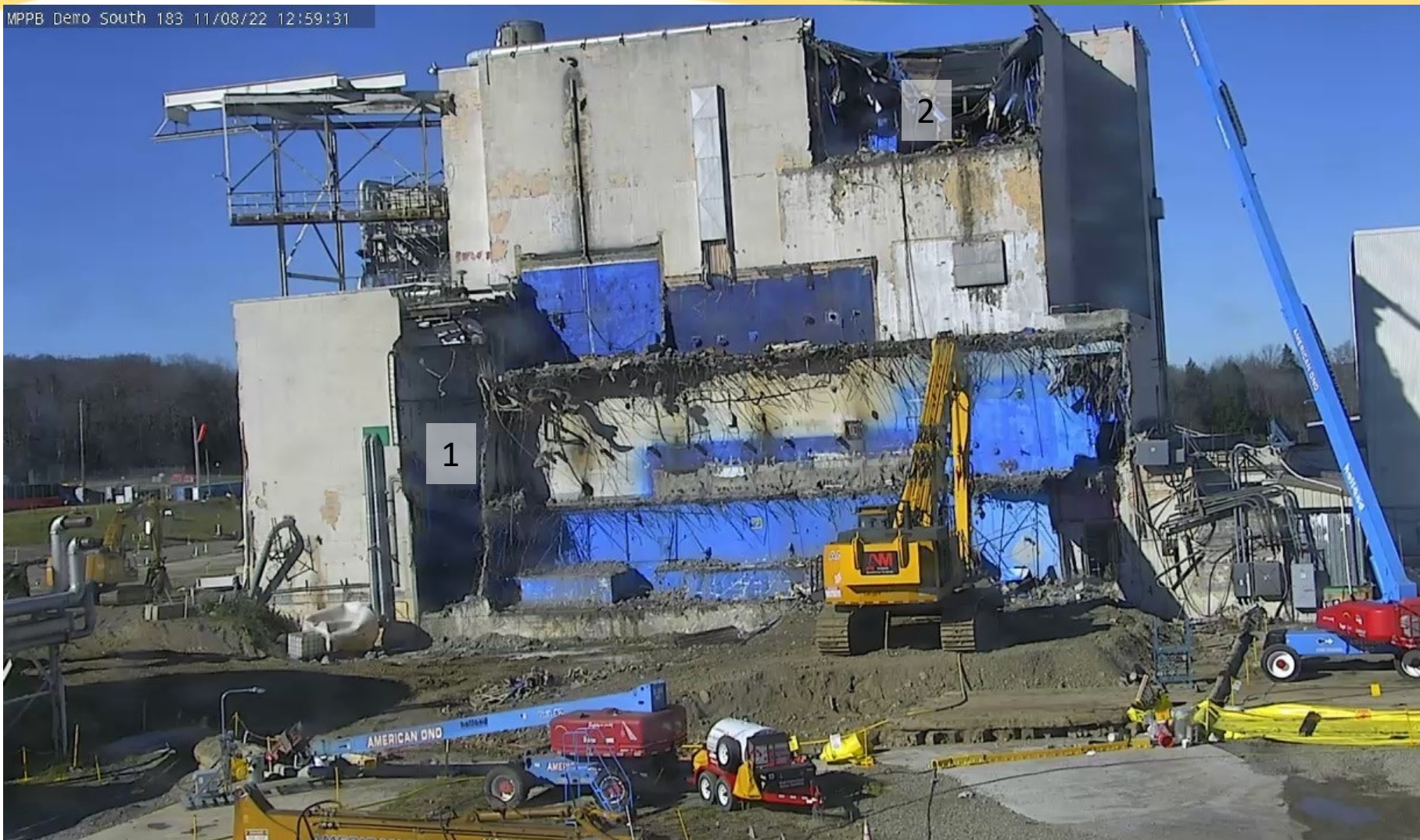
South Stairwell (1) removed and started Extraction Chemical Room (2)
