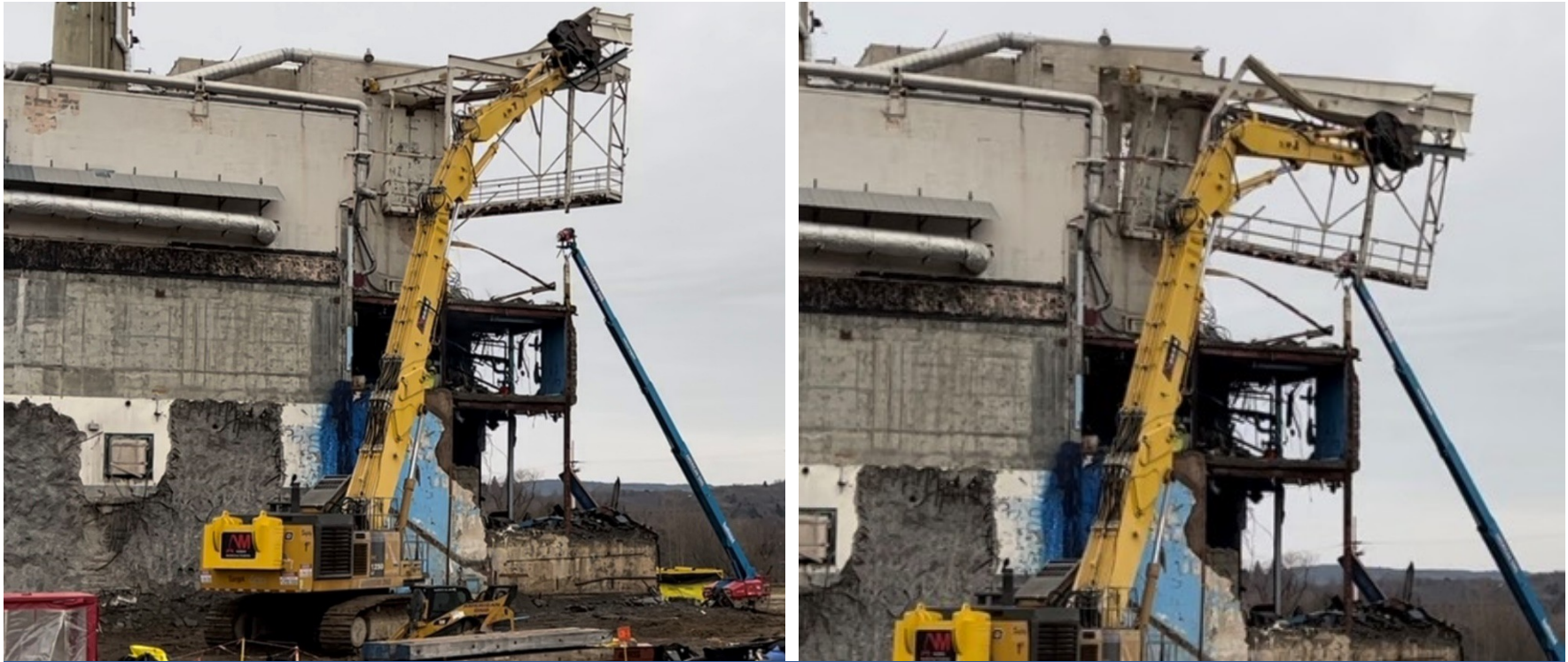
Deconstruction of Extraction Cell Monorail Crane
