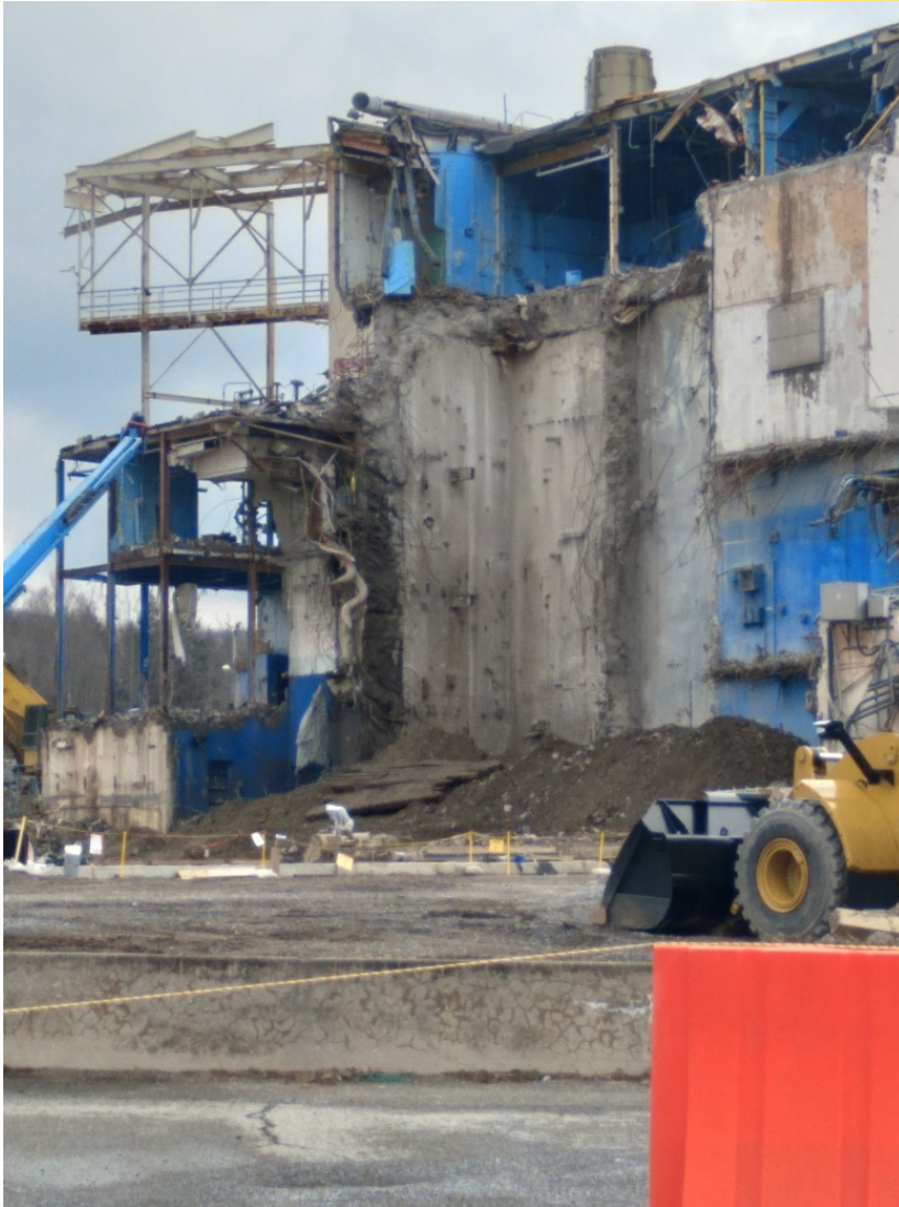
Acid Recovery Room – Off-Gas Operating Aisle (ARC-OGA) deconstruction of walls (left) and floors (right)
