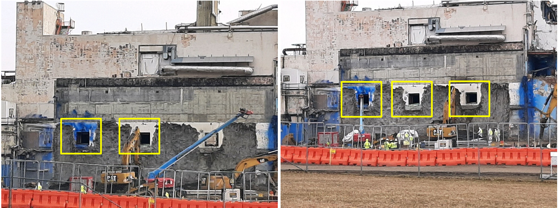
Removal of Chemical Process Cell shield windows
