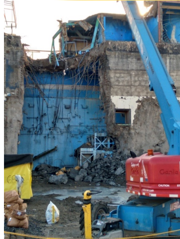
Deconstruction of Chemical Process Cell on the west side of Main Plant
