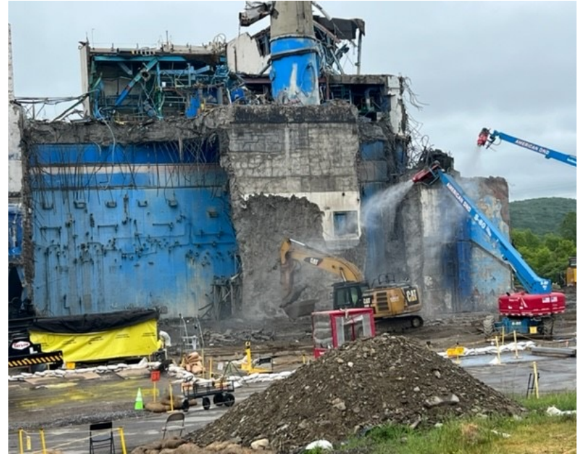
Deconstruction of Chemical Process Cell, managing the debris pile (June 12)
