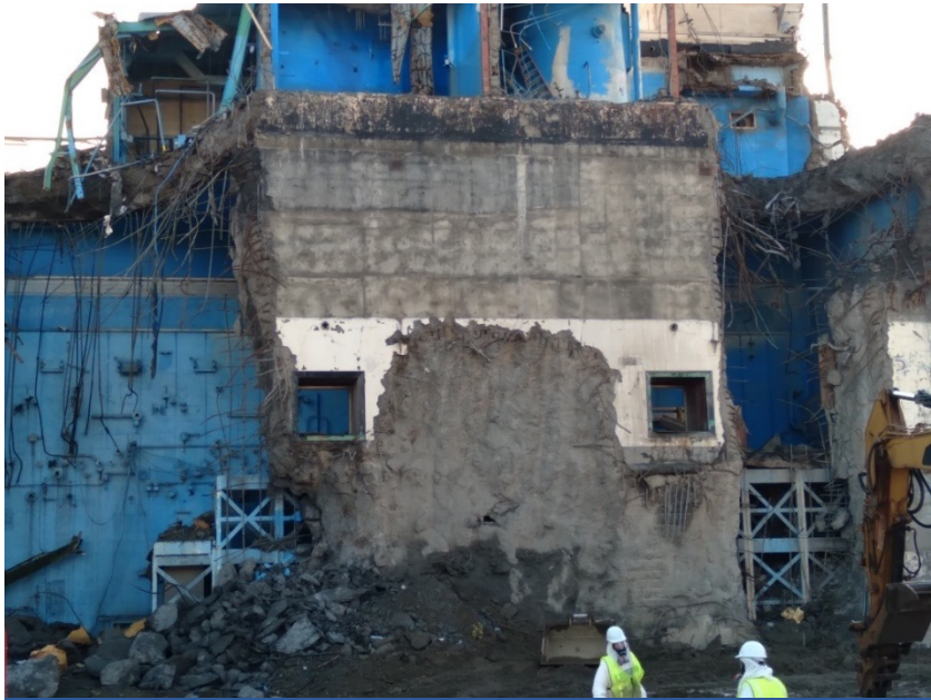
Deconstruction of Chemical Process Cell on the west side of Main Plant
