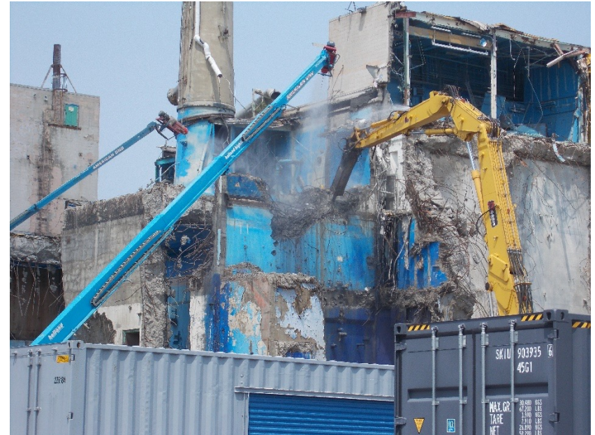
Deconstruction of Chemical Process Cell south wall (May 22)
