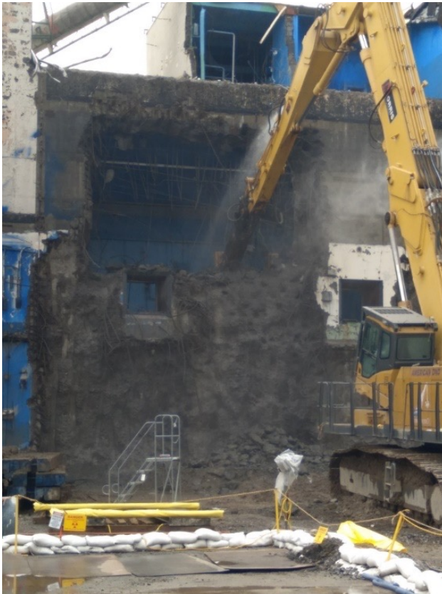
Deconstruction of Chemical Process Cell on the west side of Main Plant
