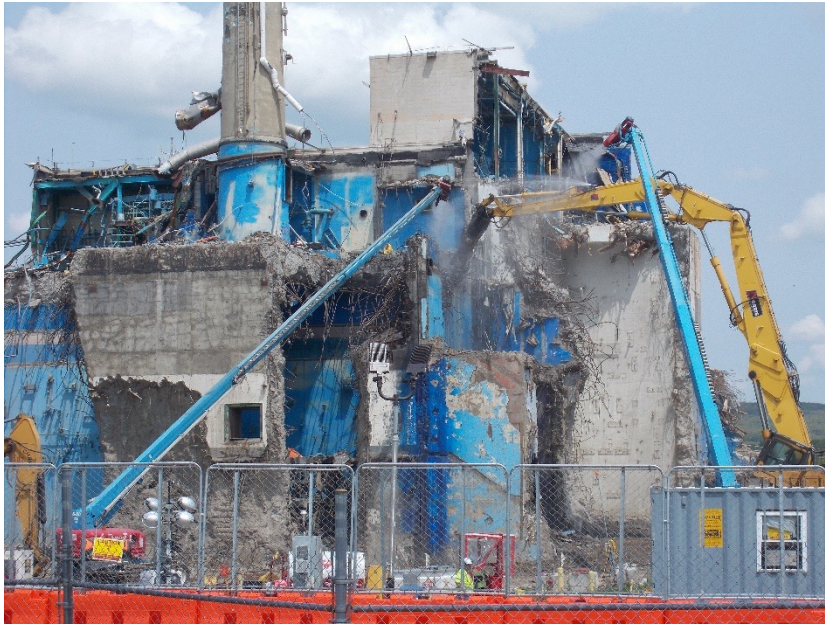
Deconstruction of Chemical Process Cell south wall (May 22)
