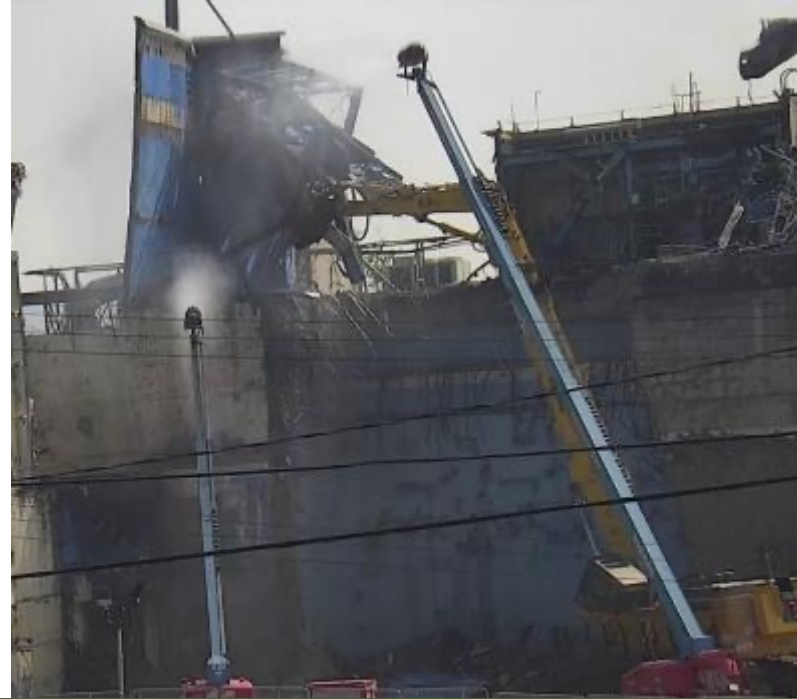
Deconstruction of the Chemical Process Cell Penthouse Enclosure
