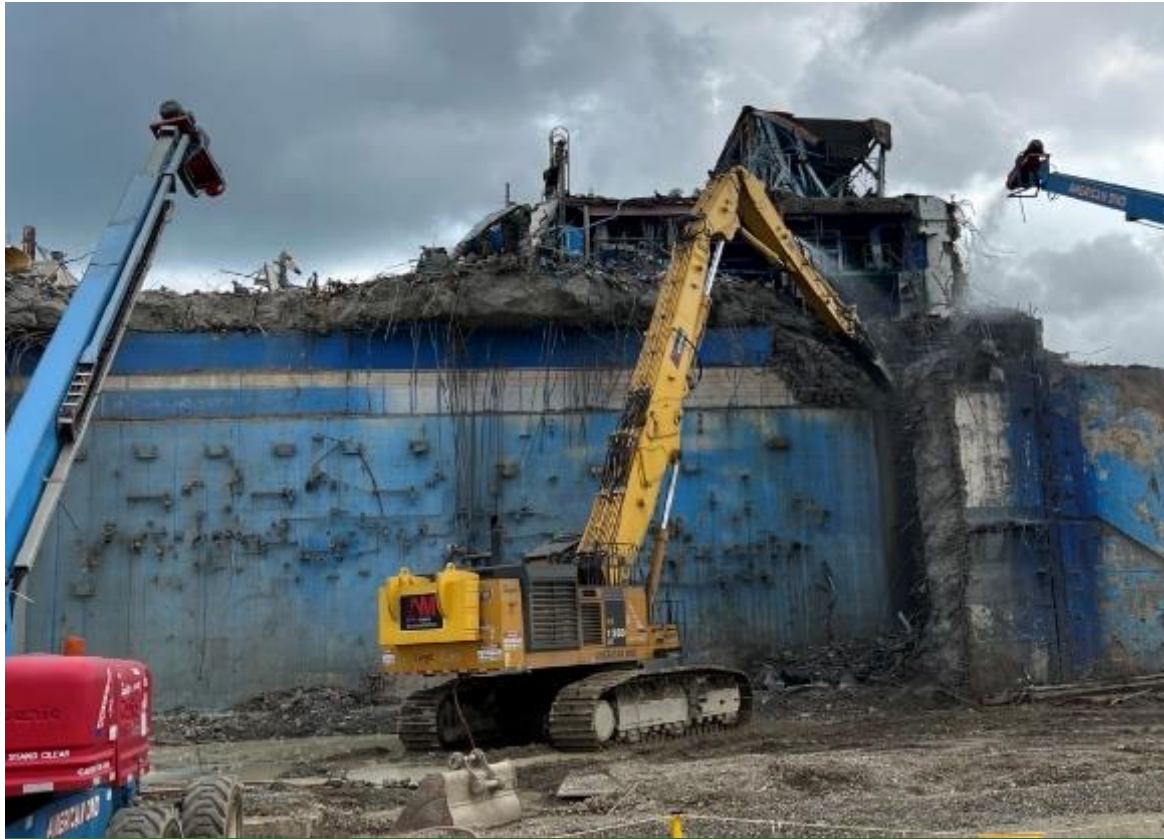
Chemical Process Cell Upper East Wall Removal
