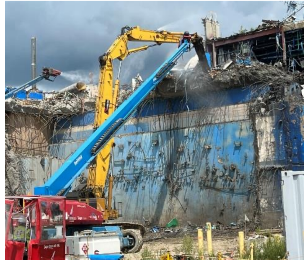
Chemical Process Cell Upper East Wall Removal
