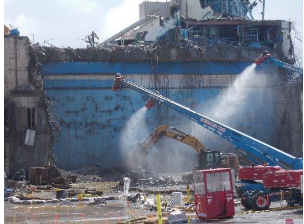
Waste Loadout of Demolition Debris
