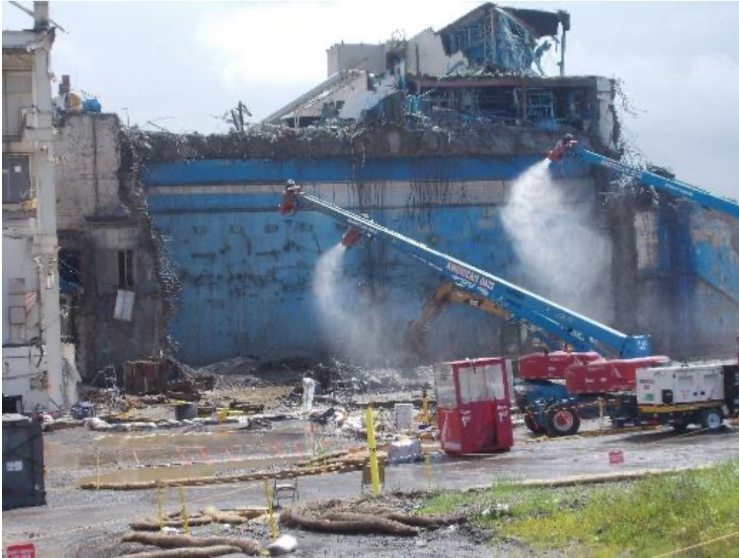
Waste Loadout of Demolition Debris
