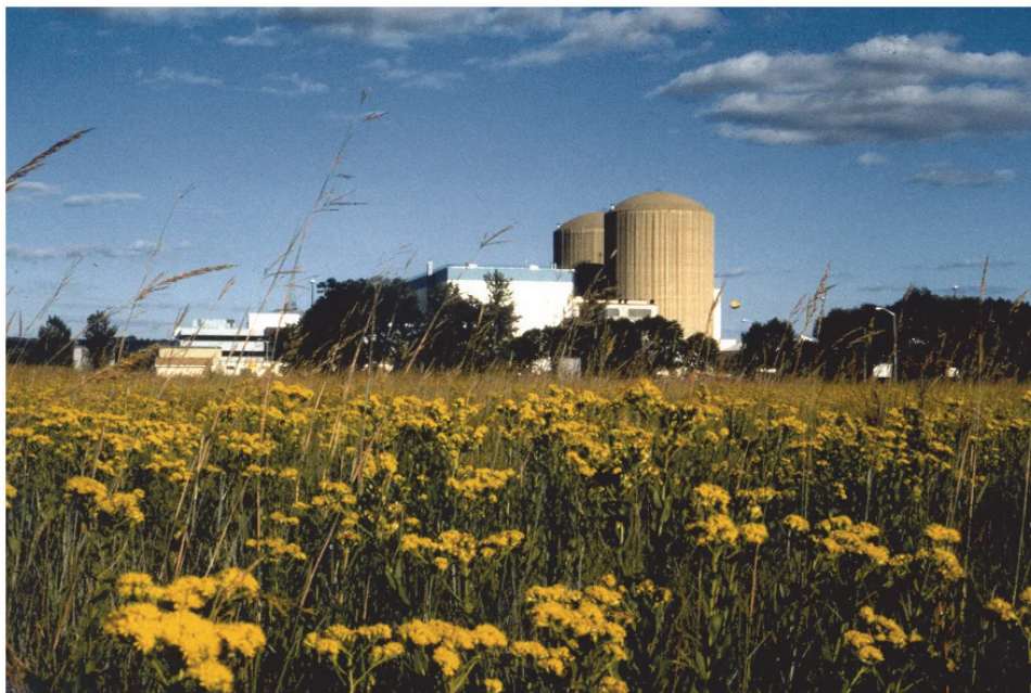
Prairie Island nuclear generating plant, units 1 and 2, near Welch.
