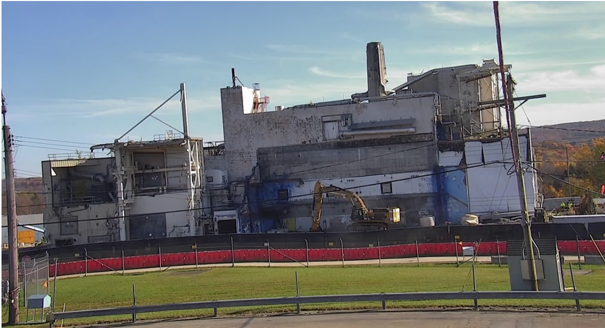
Main Plant West Wall Before Deconstruction (June 2022)
