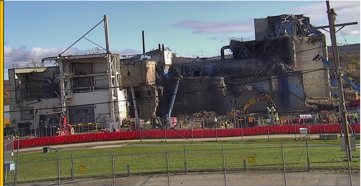
Main Plant West Wall After Deconstruction (October 2023)
