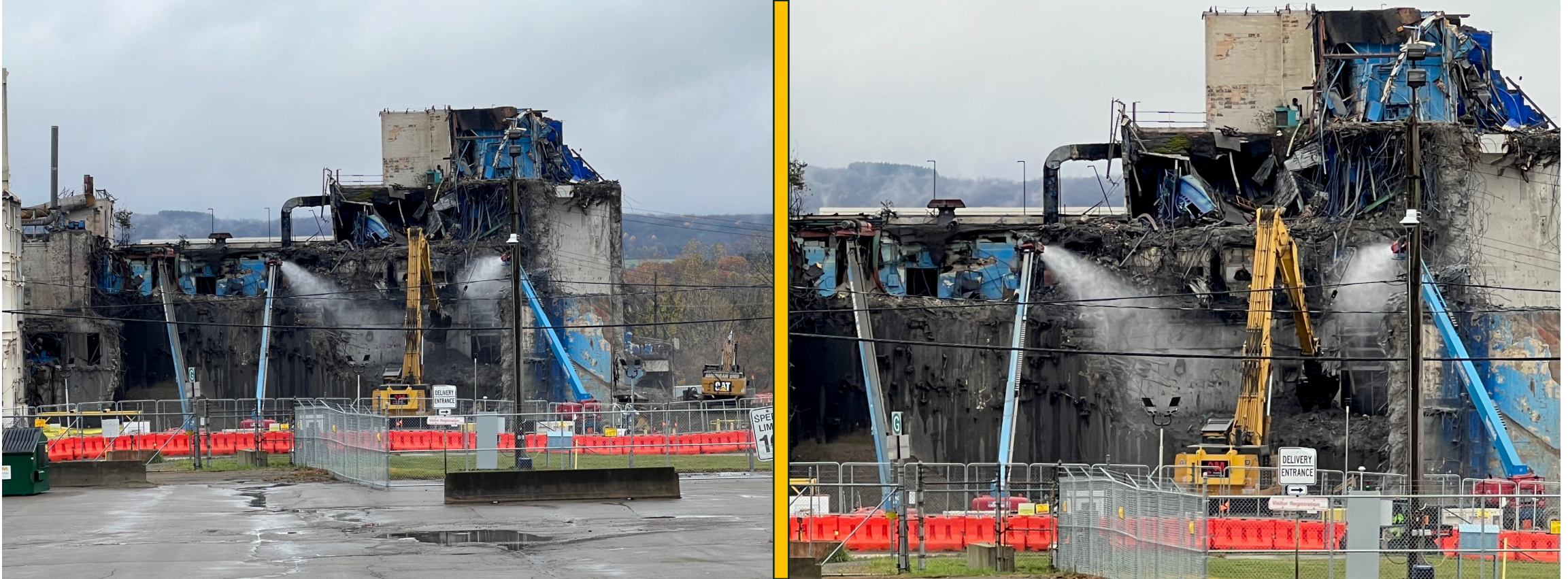
Hot Cell Deconstruction
