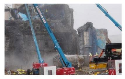
A crew from CHBWV, the contractor in the cleanup at the West Valley Demonstration Project, removes a 20-ton tank that once held high-level waste from the Main Plant Process Building. It was the first and largest of nine tanks being removed from a liquid waste cell of the building being demolished.
