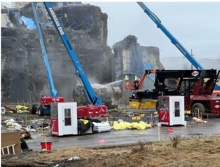
Workers at the West Valley Demonstration Project prepare a large tank for loading after removing it from a liquid waste cell of the Main Plant Process Building. (Photo: DOE)
