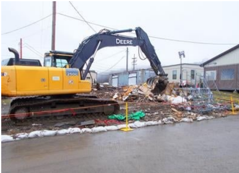
Crews demolish the old guardhouse at the West Valley Demonstration Project.
