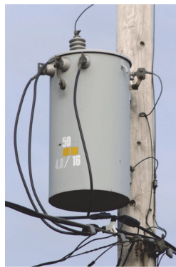
Distribution line with transformer
