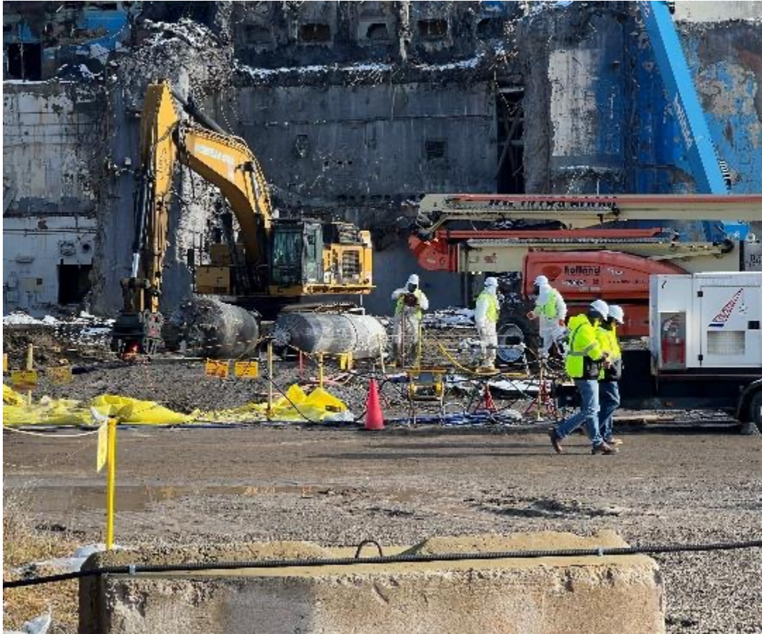
Liquid Waste Cell Tank 3D-2 and 7D-14 removed from Main Plant and prepared for loading
