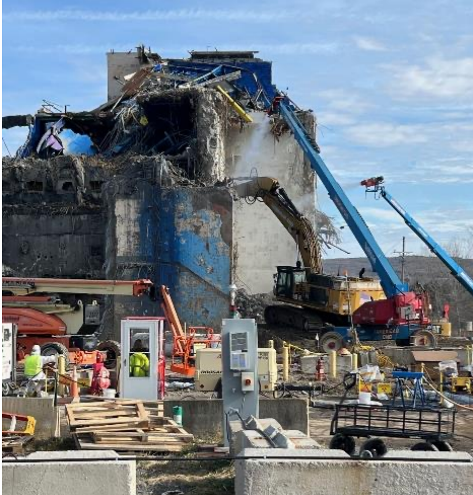
Deconstruction of Extraction Cell #1 north wall
