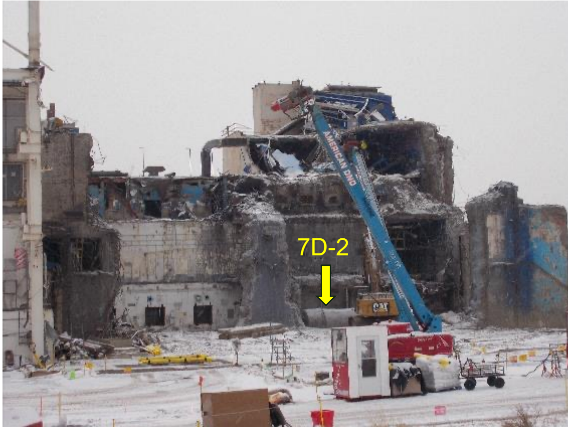
Liquid Waste Cell tank removal (7D-2)
