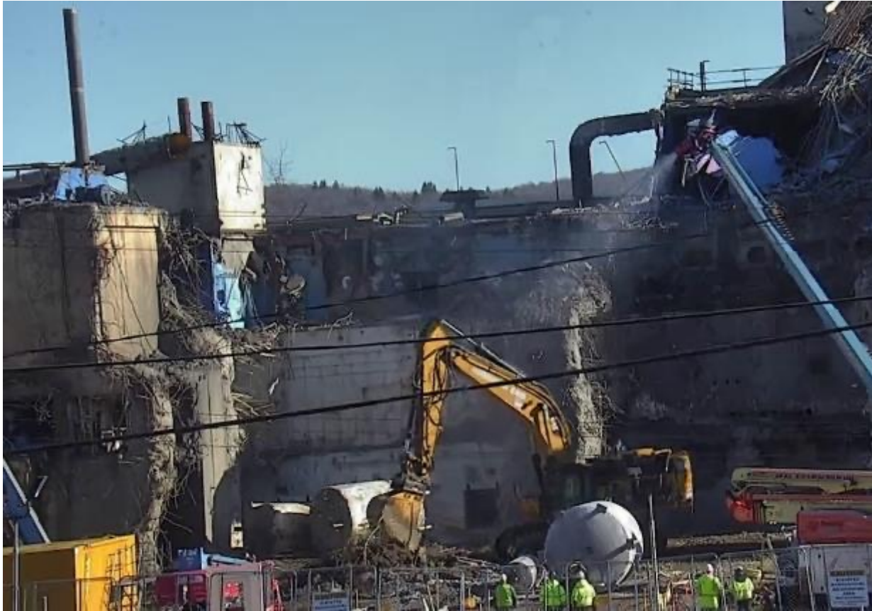
Liquid Waste Cell tanks removed, and one being loaded
