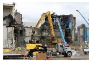
An operator uses a hydraulic grapple to safely remove and package a sampler system into a specialty shielded container for offsite disposal at the West Valley Demonstration Project.
