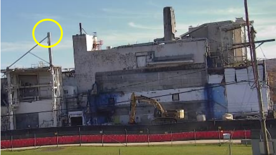
Main Plant west wall before deconstruction (June 2022)
