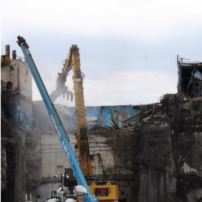
Removing debris on the west side of the Main Plant with a grapple attachment
