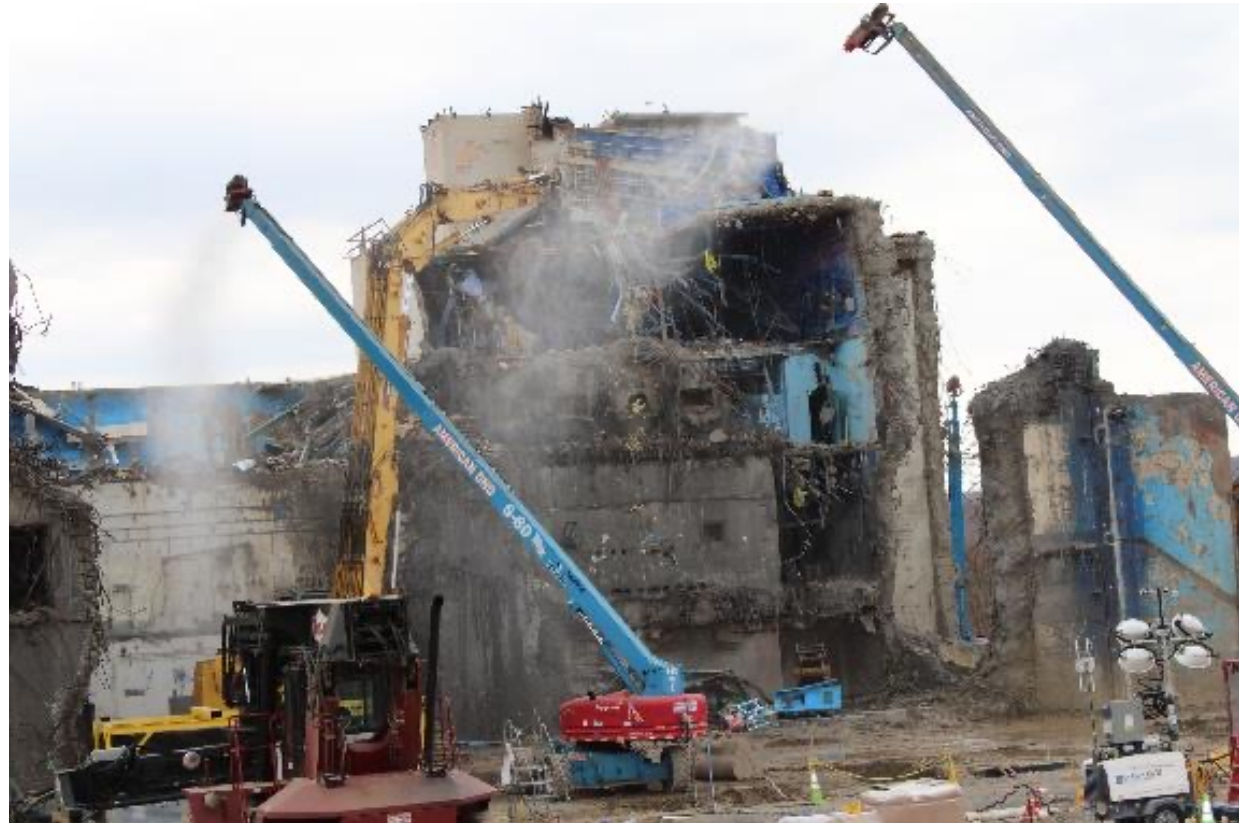
Removing debris on the west side of the Main Plant with a grapple attachment
