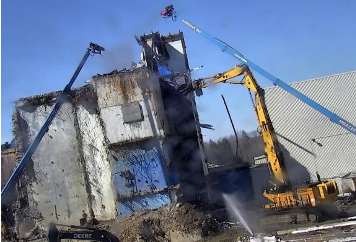
Deconstruction of the East Stairs
