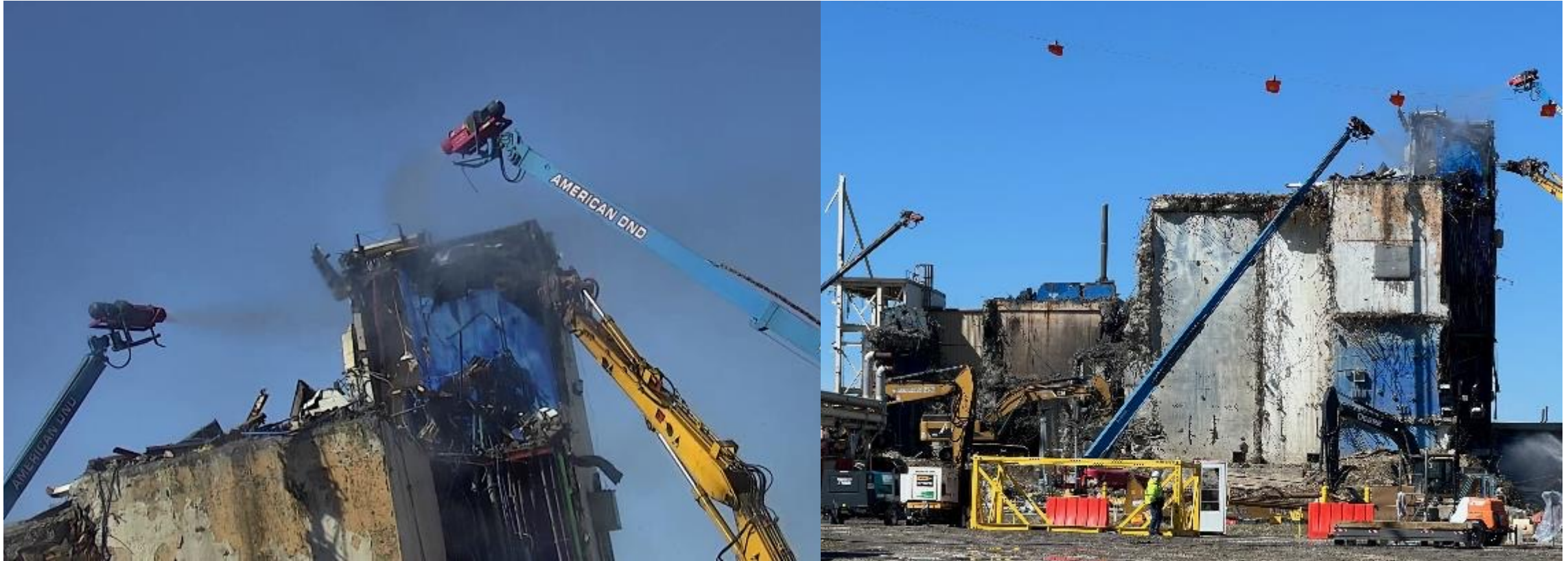
Deconstruction on Extraction Chemical Room upper east wall
