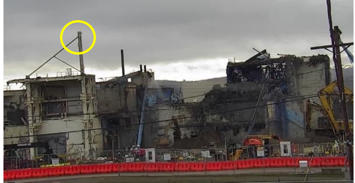
Main Plant west wall (April 2024)
